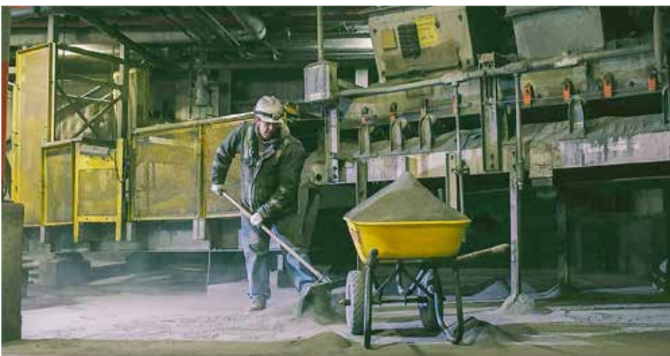
Some contractors only address the effects of conveyor inefficiency, while others offer solutions to remedy the root causes of inefficiency.
