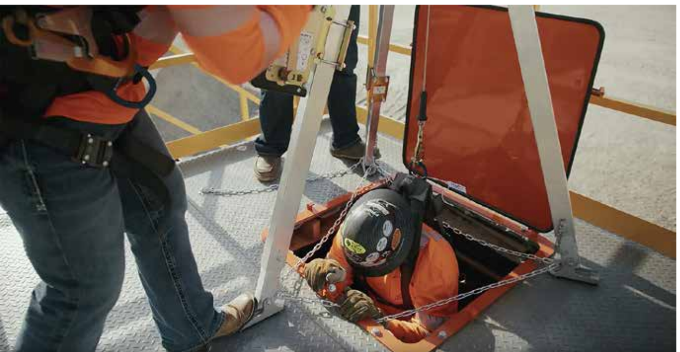
Confined space entry requires specific training since it is one of the most dangerous activities in bulk handling.
