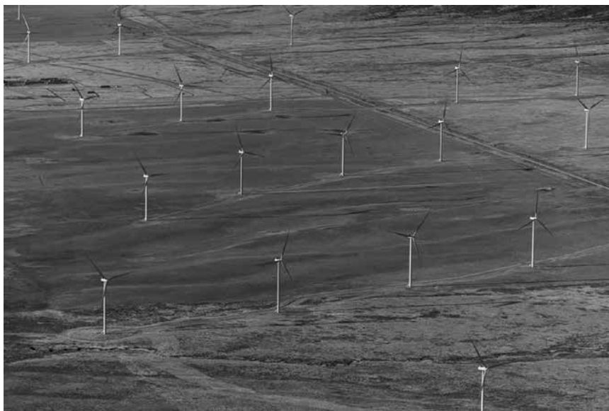
The Pryor Mountain wind farm just south of Crow Agency produces 240 megawatts of power at around 5 cents. A wind farm can generate power for 3 to 6 cents per kilowatt hour. BEN ALLAN SMITH, Missoulian.
