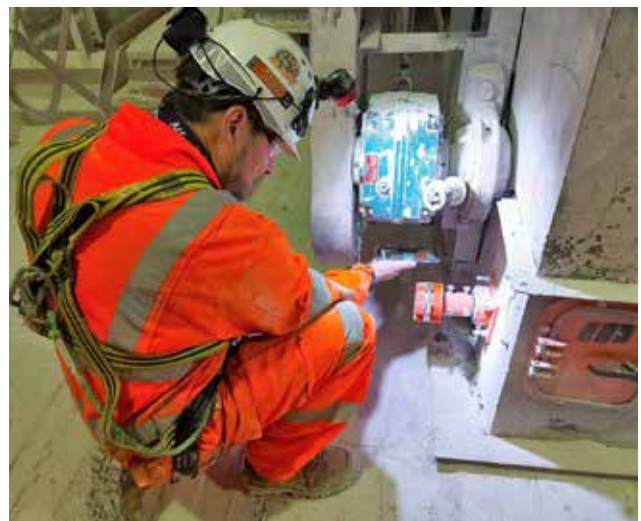
Once the central Gateway is installed and powered, each N2 ® PI can be fitted and paired in just a few minutes.
