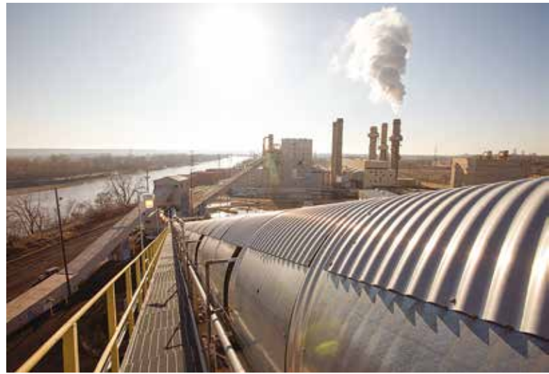
Enclosed conveyors reduce exposure to wind with fewer dust emissions leaving the site.
