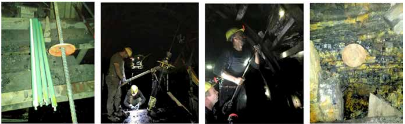
Figure 9: Typical images of the stages of RBR installation
