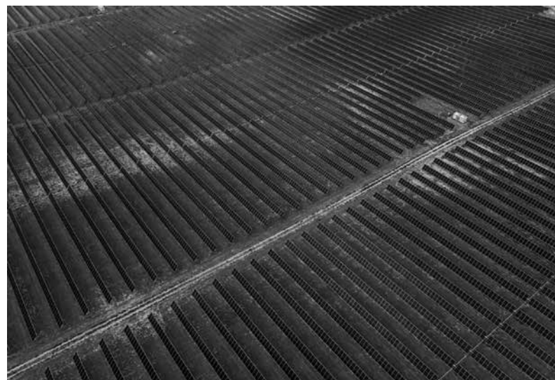
A solar farm north of Billings in August. Regionally, the solar and wind farms between Pryor Mountain and Billings now produce more day after day than Colstrip does. BEN ALLAN SMITH, Missoulian
