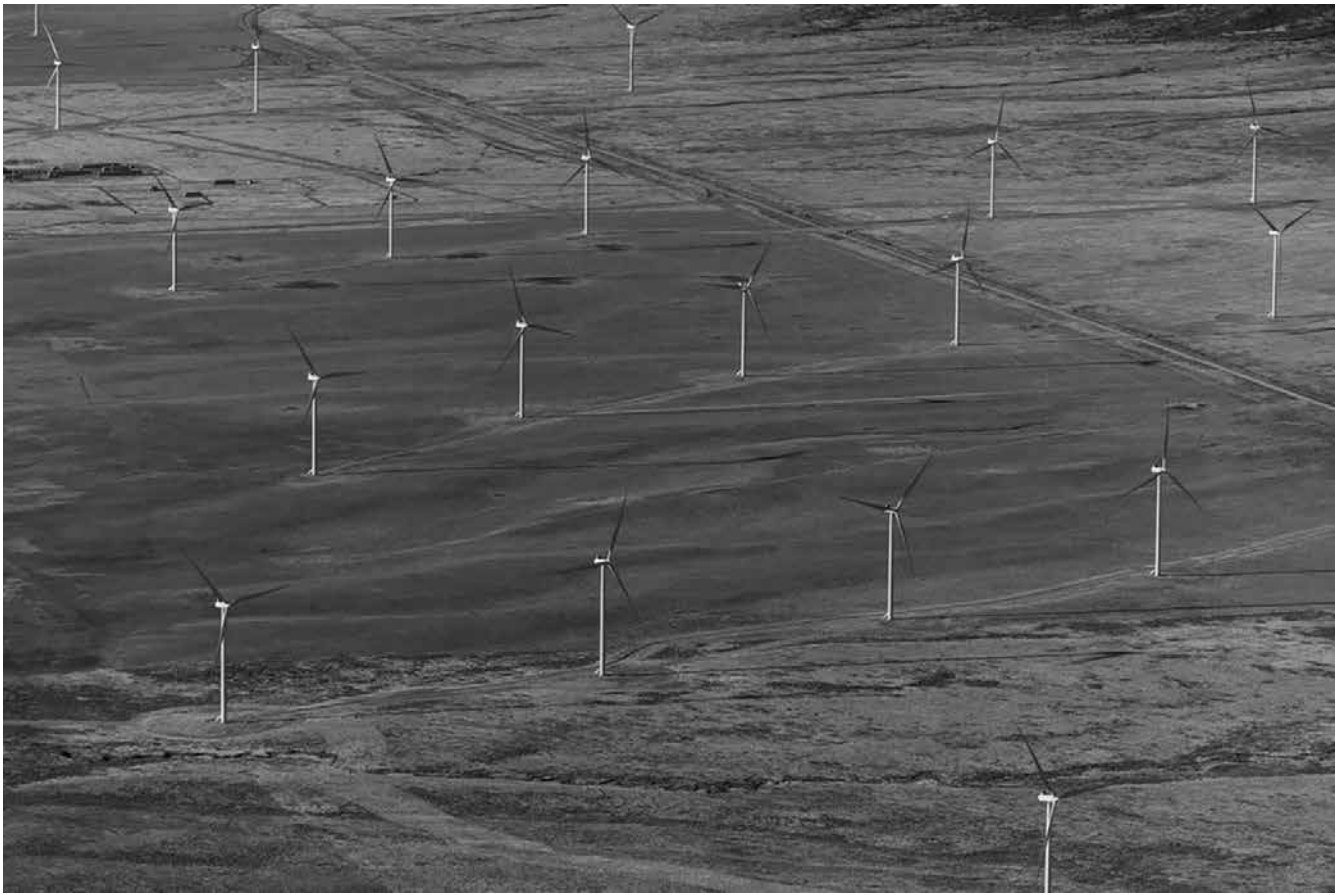
The Pryor Mountain wind farm just south of Crow Agency produces 240 megawatts of power at around 5 cents. A wind farm can generate power for 3 to 6 cents per kilowatt hour. Credit: BEN ALLAN SMITH, Missoulian
