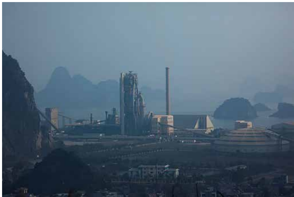
A power plant in Mao Khe City, Vietnam.
