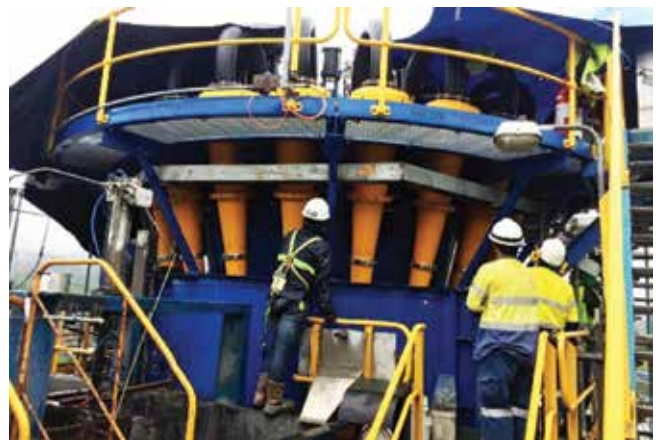
Cavex® 400CVX10 hydrocyclone cluster at Didipio Project gold and copper mine.
