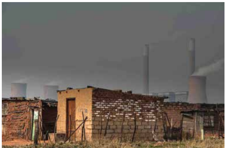
Duvha power station near Emalahleni: Eskom's strategy is to procure coal for the life of its power stations, or the life of coal-mining reserves. Photo © Mujahid Safodien/courtesy Life After Coal.
