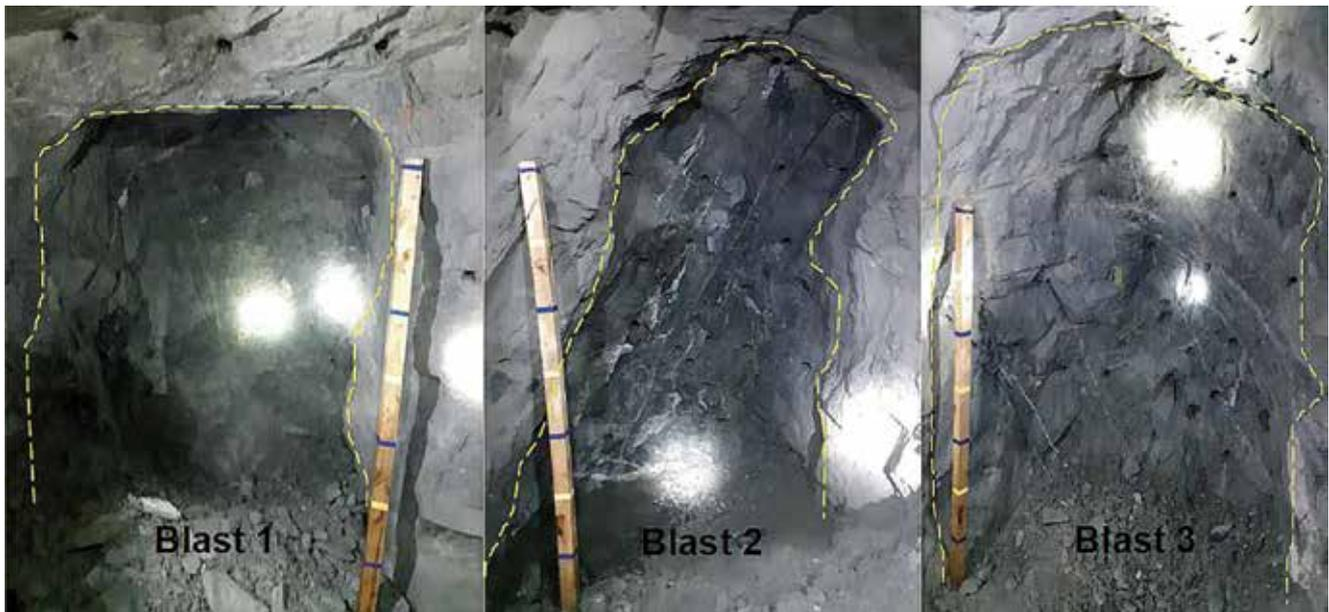
Figure 9: Compared visual results of the 3 blasts.
