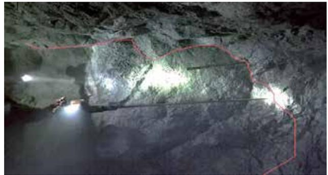
**Figure 3:** Result of blasting at the Mina La Palmera, showing the overbreak profile.
