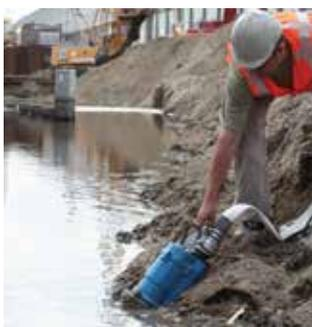
Theoretically, the number of pumps that can be operated in series is unlimited. Significant capacity losses are not to be expected. With two identical pumps, the achievable distance performance is roughly doubled. However, the flow rate remains the same. If one wanted to increase this, parallel operation of the pumps is necessary or the use of larger models.
