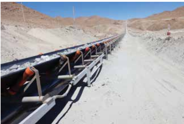
KUMERA powered overland conveyor in operation in Chile.
