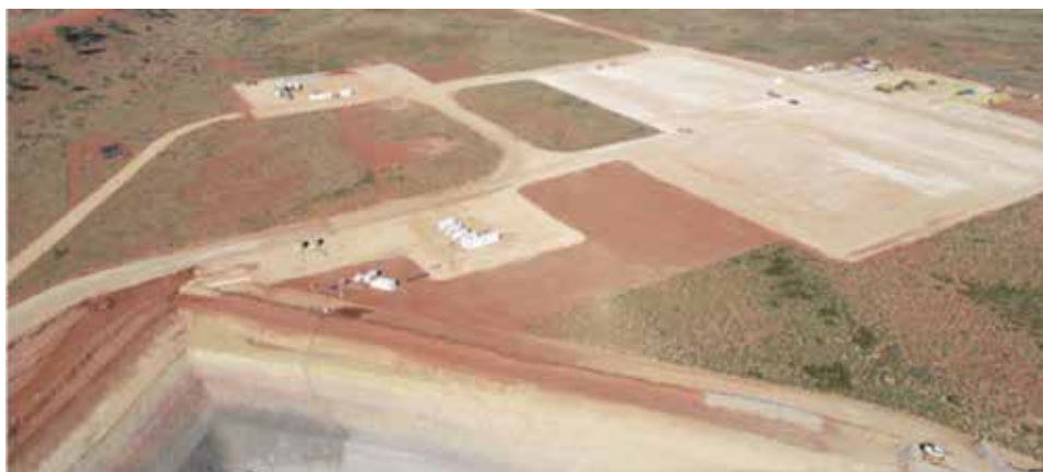
An aerial shot of the Havieron boxcut.
