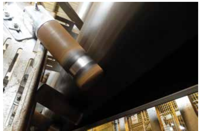
For the entire project, BEUMER Group was able to ensure that the iron ore is transported safely and quietly, without disturbing the residents or disrupting the surrounding nature.
