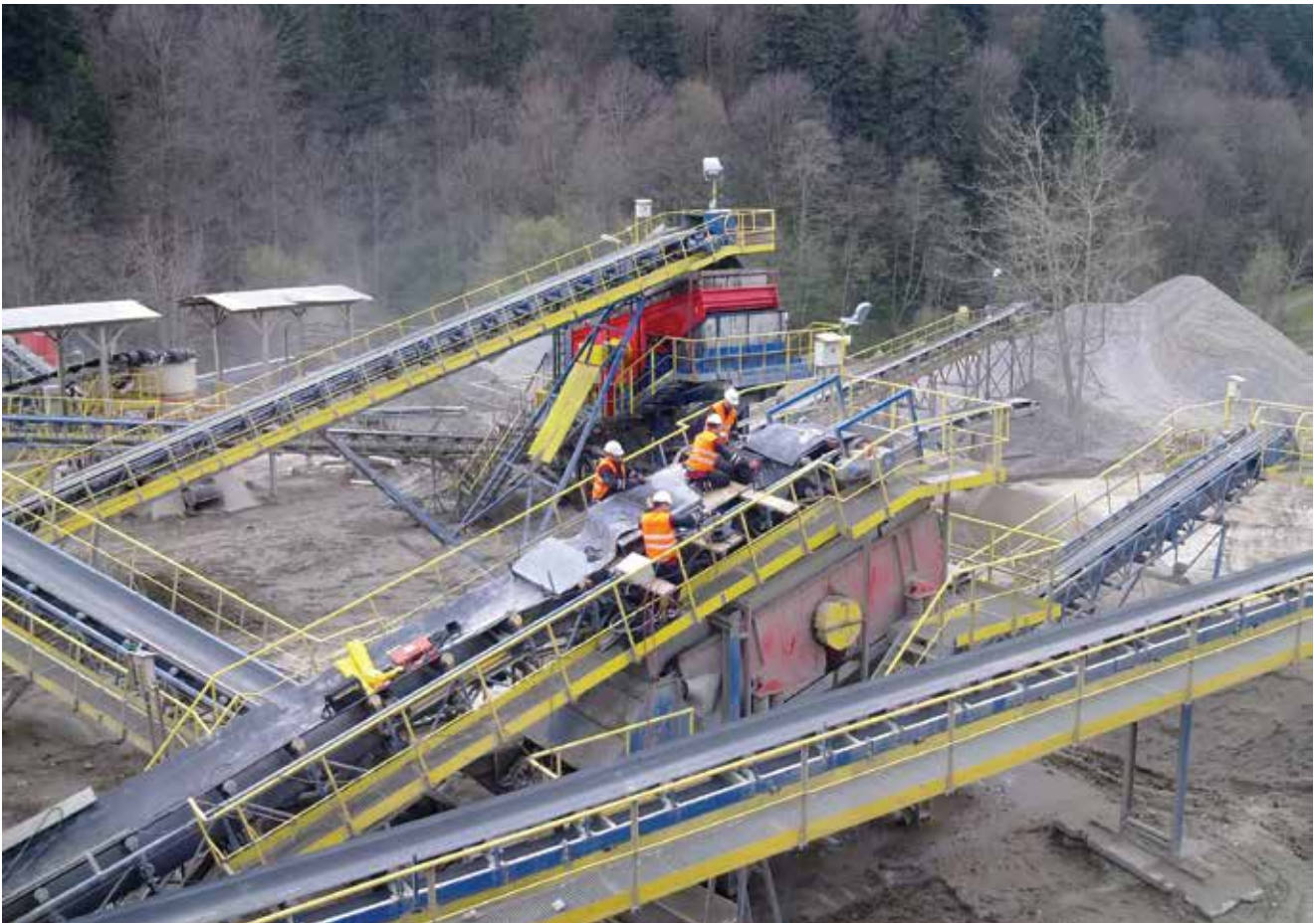
The cost of making the splice is a small fraction of the cost of a system shutdown.
