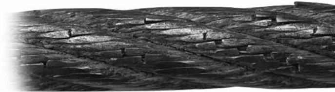
“SQUARED ENDS” > Typical example of breaks due to fatigue.
