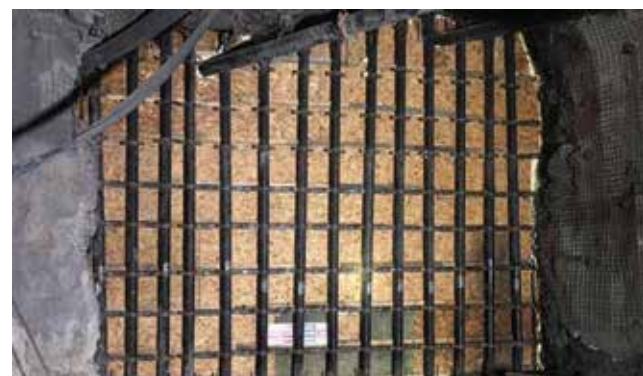
Figure. 1: Ventilation stopping.
