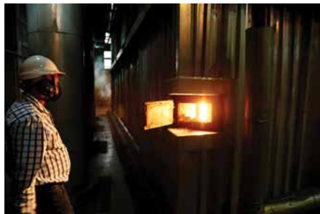
The coal furnace used to power a turbine at the Komati Power Station in Mpumalanga.
