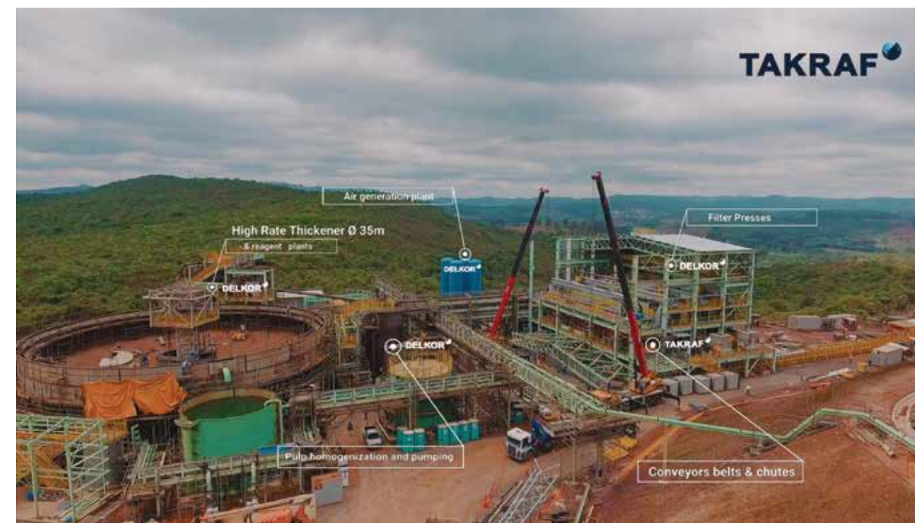
DST system under construction for the safe and effective handling of iron ore process tailings recently supplied by TAKRAF Brazil to Mineração Usiminas. Source: TAKRAF
