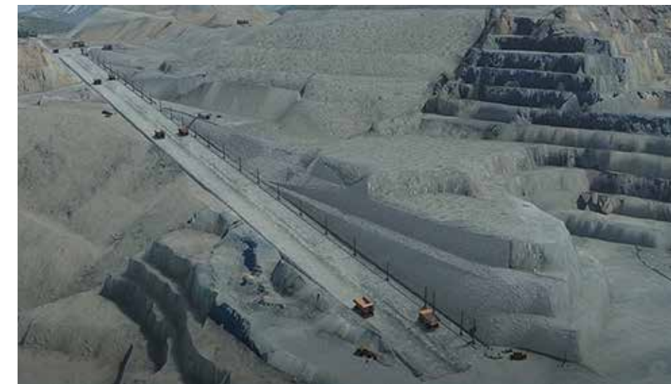
Four Komatsu hybrid trucks at a time will be able to climb, via electric trolley assist, up a one-kilometre hill from the pit at Copper Mountain mine near Princeton to the operation's primary crusher. (Visualization courtesy of Copper Mountain Mining Corporation).
