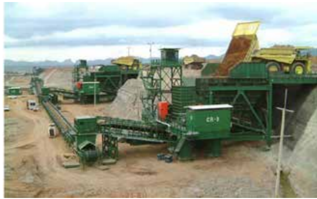
Figure 6: Semi-Mobile In-pit Crushing and Conveying systems (Source: Sandvik Mining and Construction).
