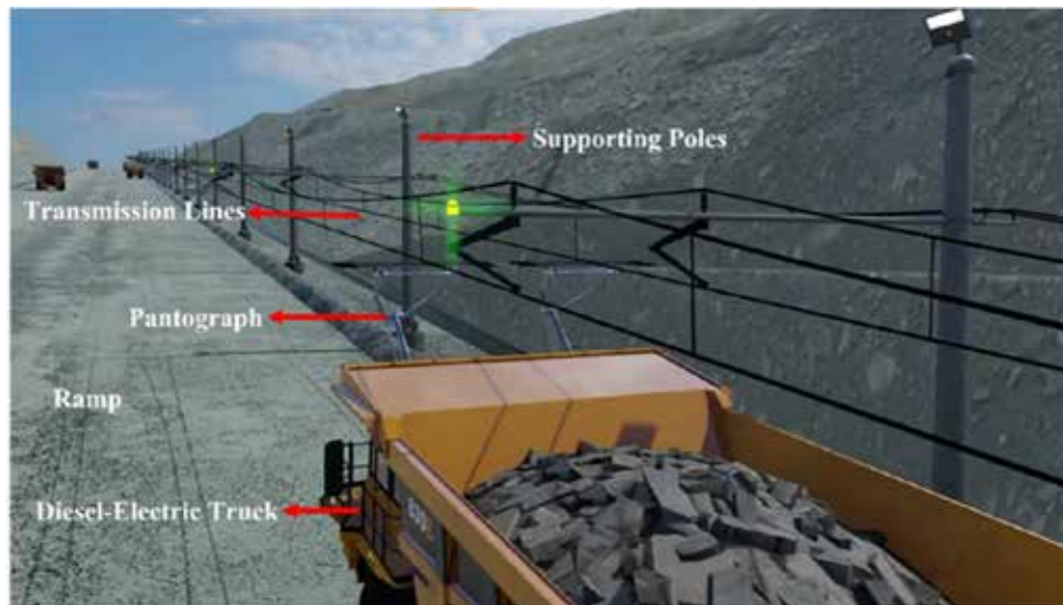
Figure 12: Truck with Trolley Assist capability operating on ramp (Source: ABB).
