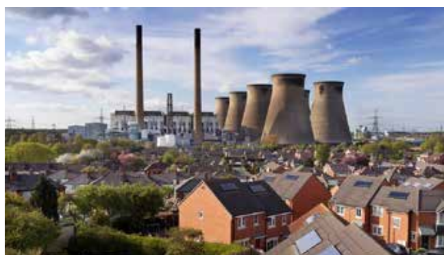
One of the UK's defunct coal plants in Ferrybridge, West Yorkshire, is being turned into a battery energy storage system (Credit: Getty Images)
