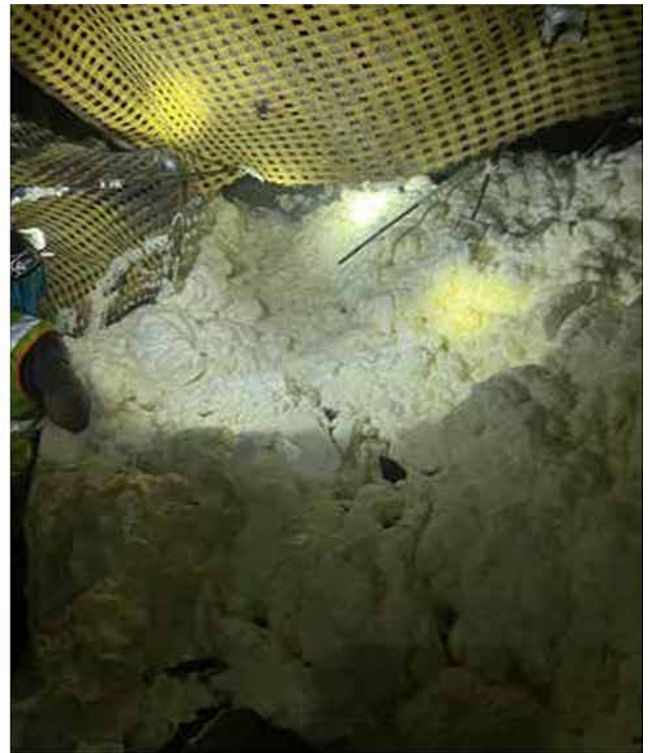
Ultra-X Foam is a two-component grout that is intended for, strata consolidation, coal face reinforcement, and large or small cavity filling.
