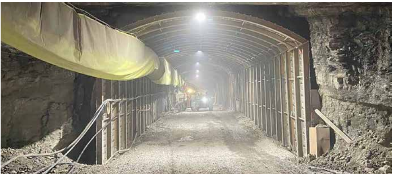
J-SEAL is a specialized foaming cement which can be used for backfilling behind steel sets or other general backfilling applications in coal or hard rock mining.
