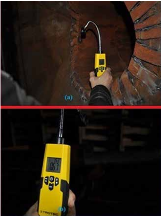
Figure 3: Air velocity measurements, (a) air inlet clearance (5.39 m/s); (b) air velocity inside the gallery (0.67 m/s).
