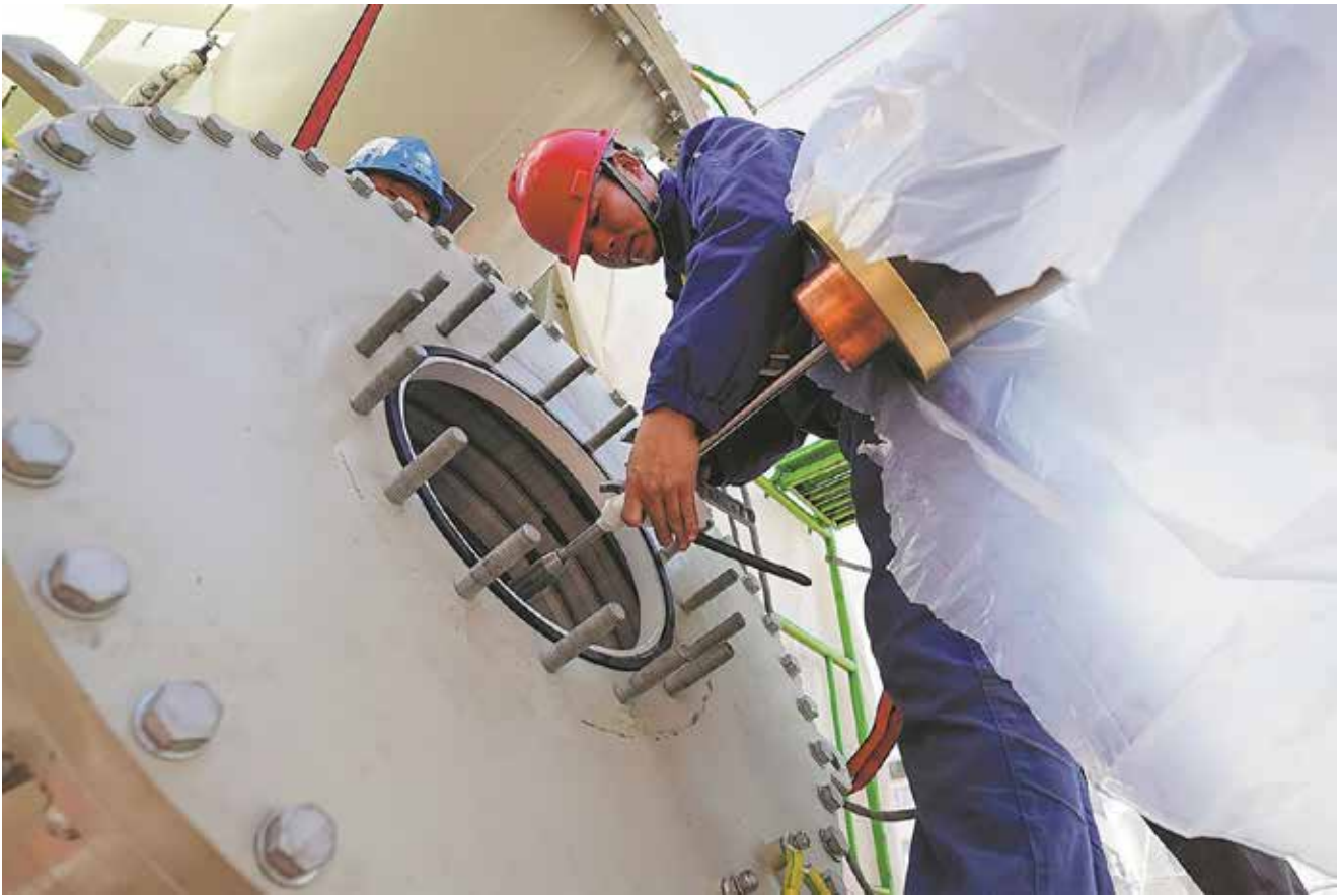
A worker installs a spare rectifier transformer bushing at Balikun converter station in Hami, Xinjiang.
