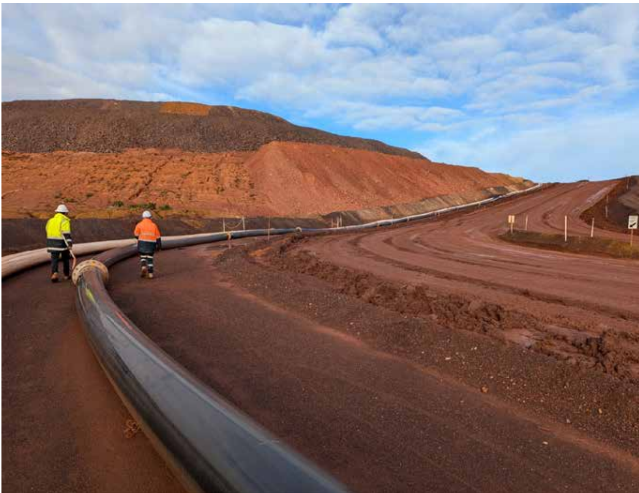
Formed flanges and face-to-face sealing of Arterra™ UHMWPE pipelines ensure smoother connections, reducing turbulence and wear.
