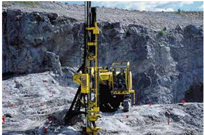
Surface drilling rig
