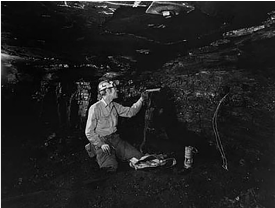
Loading a drill hole underground
