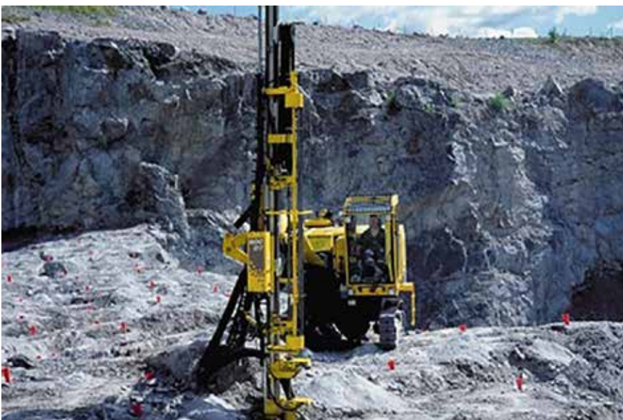
Surface drilling rig
