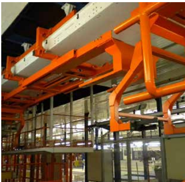
Overhead mining conveyors
