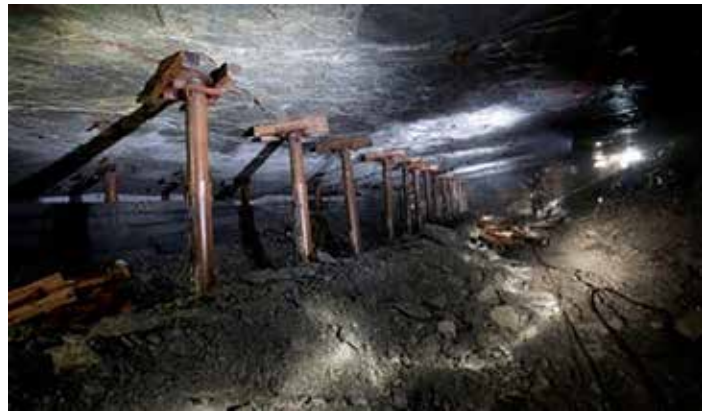
Wooden Support Beams
