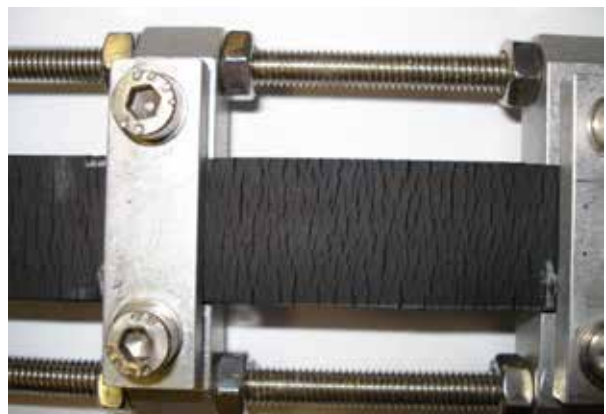
The damage caused by ozone and ultraviolet exposure is considerable.
