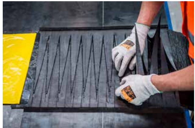
A finger splice is stronger and more reliable.
